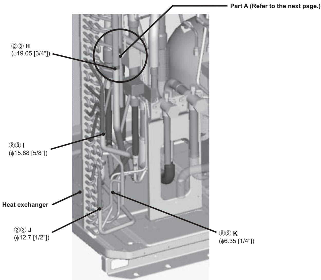
\* After removing Solenoid valve block ASSY
